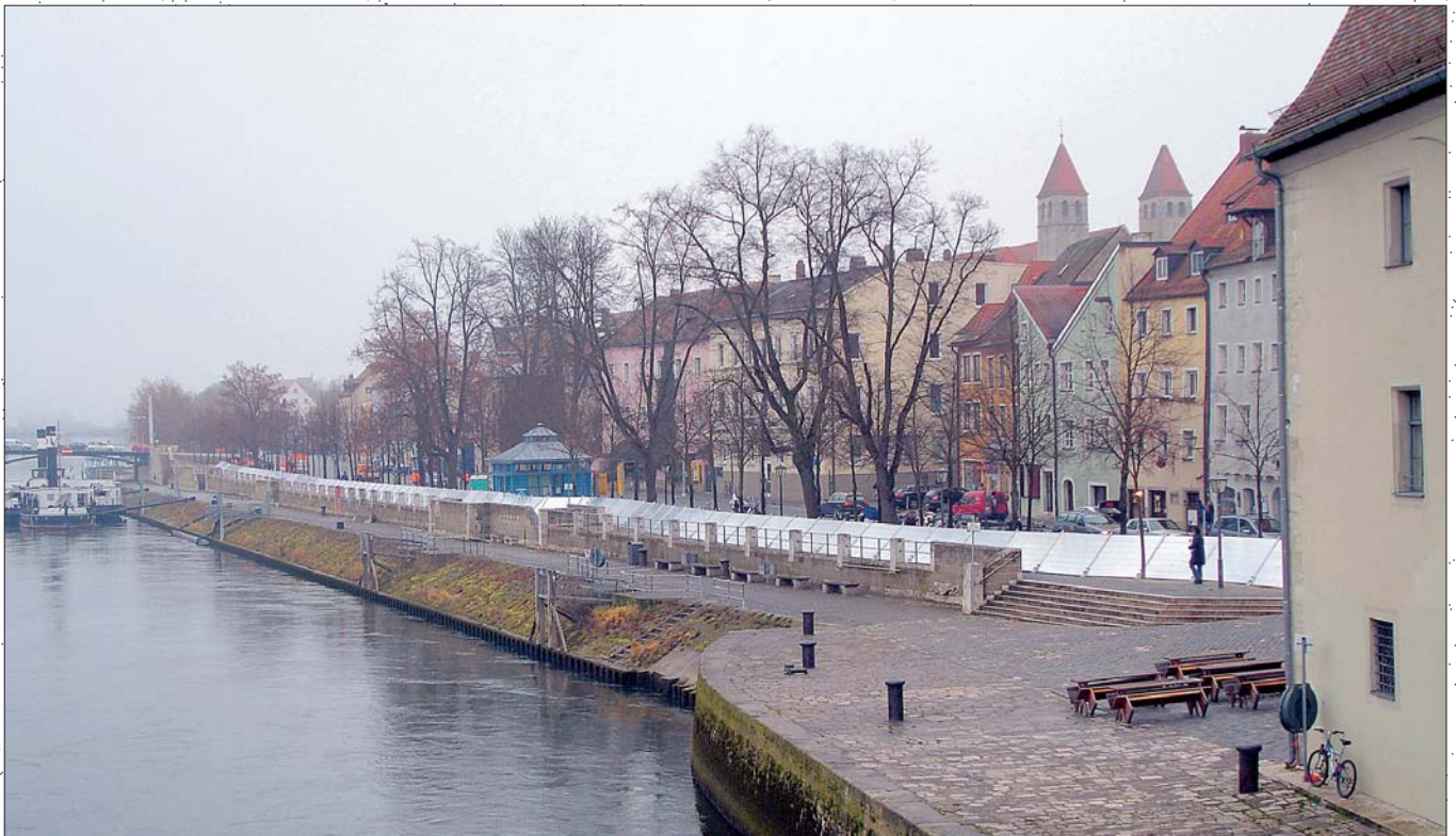
View from the Steinernen Bridge of the defence line on Thundorferstrasse
