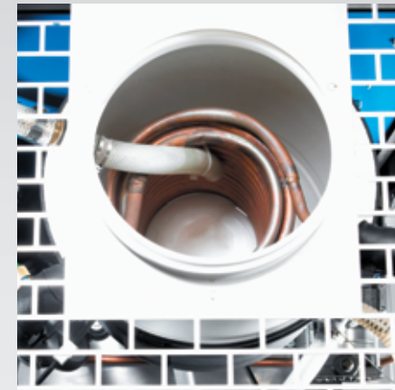
Copper coil evaporator inside the tank
