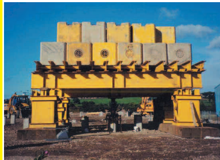
Kentledge test-frame on site at Belvedere, South London
