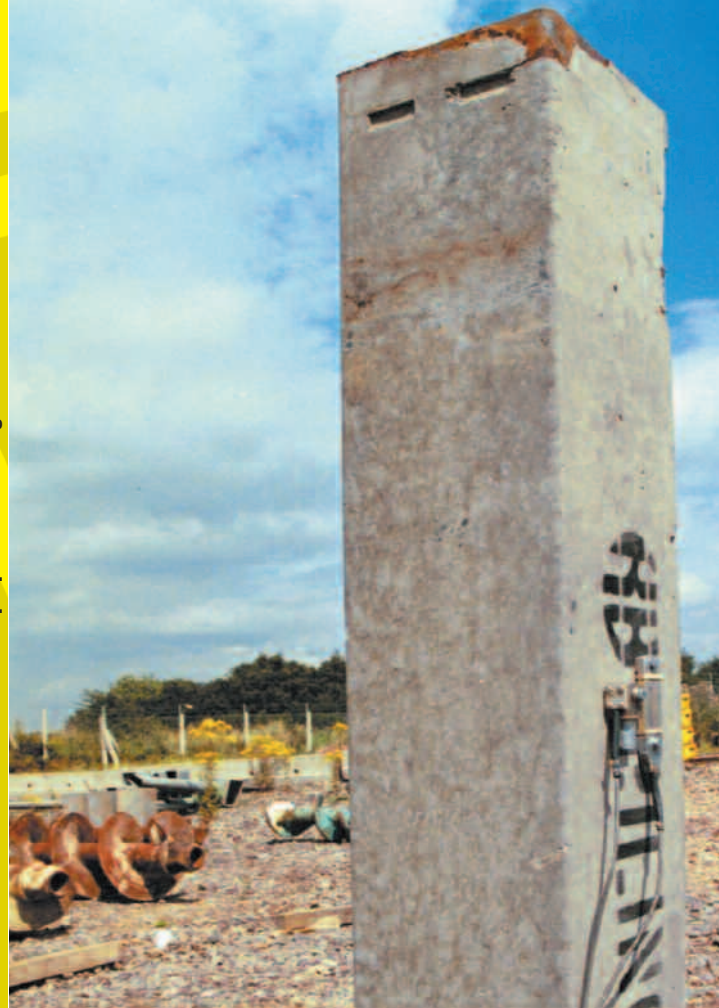
Pile prepared for testing on site
