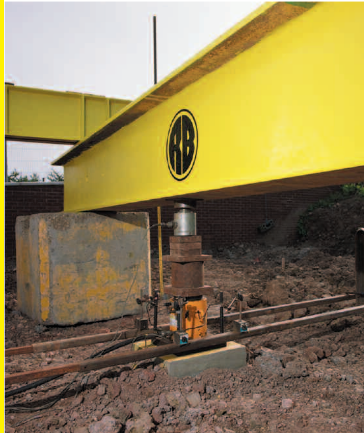
Pilehead measurement at Abingdon, Oxford
