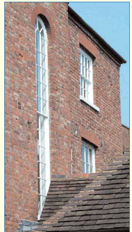
32 Church Street Tewkesbury: 1813 a remarkable elongated sash to light the staircase
