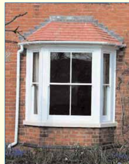
Ropewalk Tewkesbury: Victorian sash with horns
