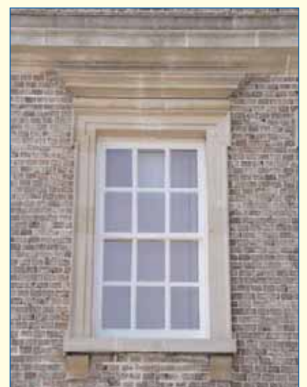
Wallsworth Hall Twigworth: window to principal elevation with classical stone surround
