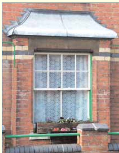
Cotteswold Road Tewkesbury: hybrid sash design typical of Edwardian houses
