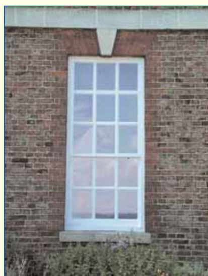
Wallsworth Hall Twigworth: mid 18th Century ovolo moulded sash window with rubbed brick lintel, stone cill and keystone
