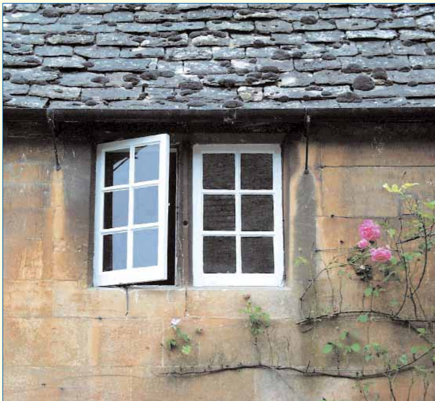
Timber casement window replacing leaded lights in a stone mullioned frame
