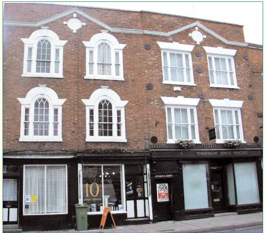
Late 18th Century curved gothic glazing bared sashes in 'Venetian' windows at 9 & 10 Barton Street, Tewkesbury with flush boxes. No 11 (right) has later 19th Century recessed tripartite sash windows
