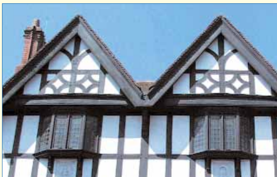
19 High Street Tewkesbury (Lloyds TSB Bank): built in 1921 in the Tudor revival style with intricate leaded light oriel windows
