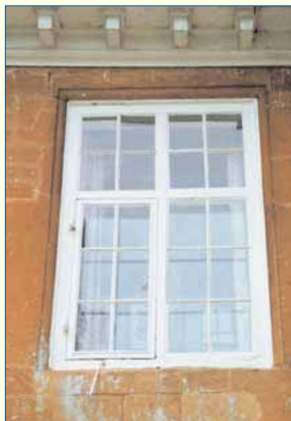
Old Rectory Dumbleton: timber cross casement early 18th Century
