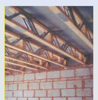
The easi-joist® floor system offers clear benefits over sawn timber and other engineered floor joist systems flooring systems. Not only does it out perform sawn timber in span and dimensional stability, the added benefits of a greater bearing area and open web system makes it easier to install for the carpenter, plumber and electrician, reducing valuable time and cost.
