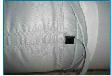
Close-up view of the tie belt
