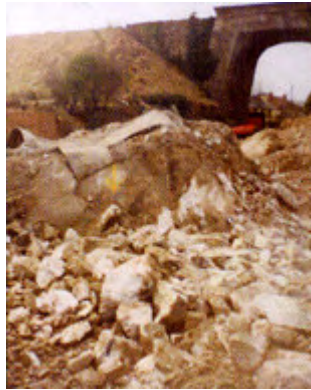
Newry Bypass - Excavation of rock adjacent to busy road.
