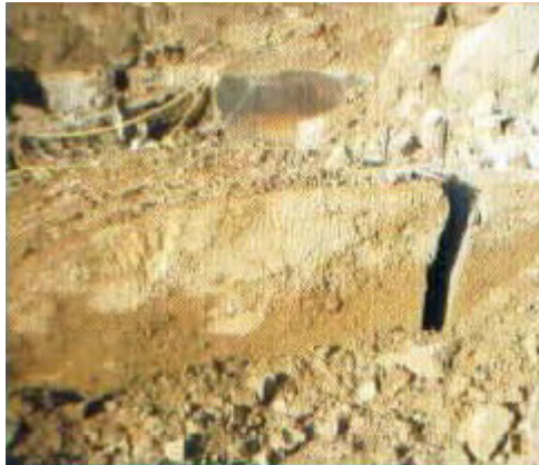
Two CARDOX Tubes split and heave a block of over 50 tonne.
