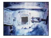
Before: Opening inspection holes reveals build-up of cement.
