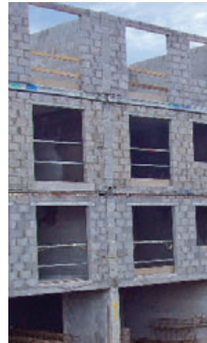
STEPOC in a multi-storey development
