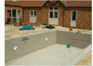
STEPOC swimming pool walls
