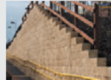
Passenger Access, Littleborough Station, Rochdale
