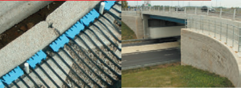
Keystone block showing grid connection
