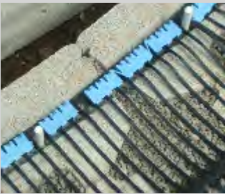
Keystone block showing grid connection
