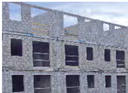
STEPOC in a multi-storey development
