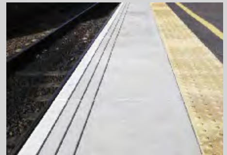
Typical platform construction
