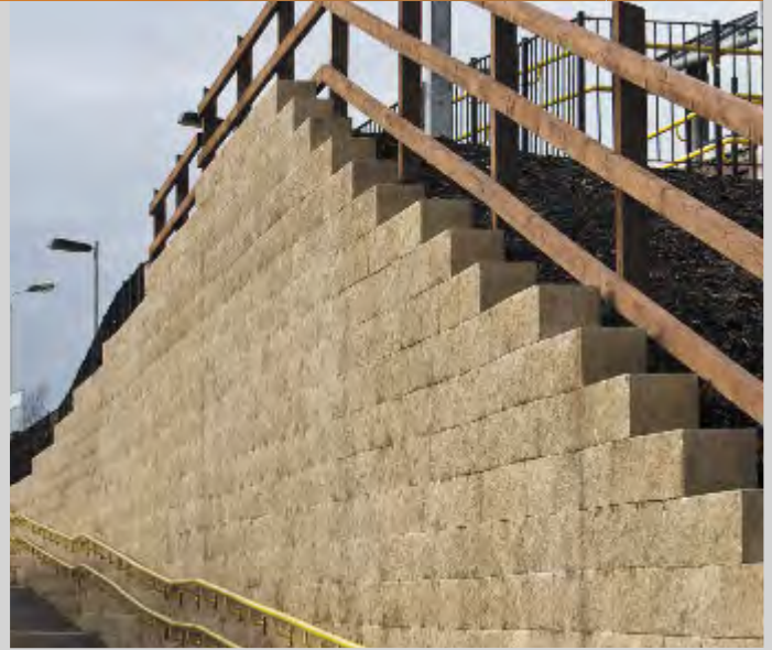
Passenger access, Littleborough Station, Rochdale
