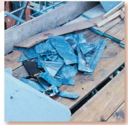
Note that old lead sheet being replaced must be removed with care. A white dust sometimes gathers on the underside and could be hazardous when disturbed. A fine dust mask should be provided and worn by <u>all persons in the vicinity</u> of such material when it is moved <u>not just those concerned with its removal</u>.
