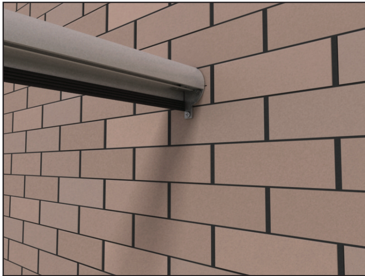
26 Drop the handrail onto the angle bracket
