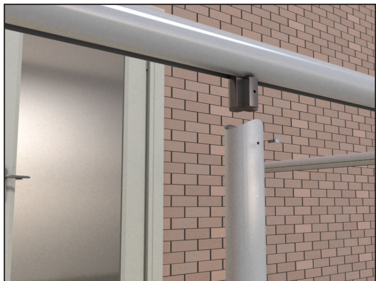
29 Fix the post into the post connector using the M5 screw provided
