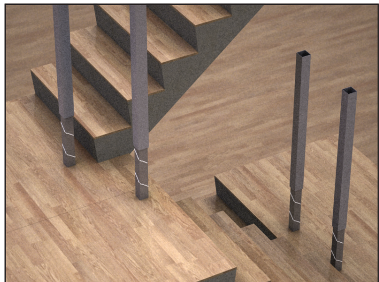
10 Slide the system covers post onto the primary posts
