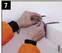
7 Firmly fasten the self-adhesive strip over the joint of the wrap
