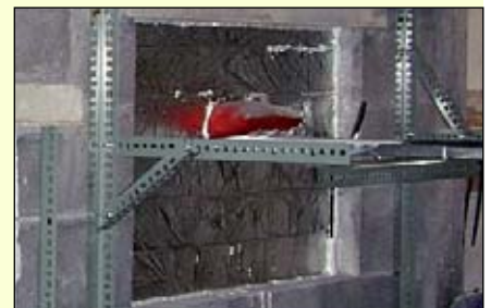
Blocks fitted into ceiling/floor penetration. Intumescent wraps A around pipes & intumescent expansion joints B over cable trays. Seal joints with intumescent acrylic mastic
