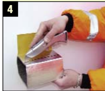
4 Cut along the marked line with a sharp knife to open up the wrap for fitting onto the trunking or ducting
