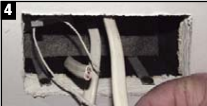
4 Once the cover is fixed, cut the string and remove from the cover
