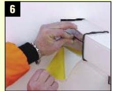
6 Whilst holding the wrap in place, remove the backing from the self-adhesive strip
