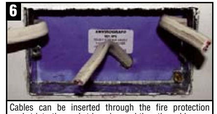
6 Cables can be inserted through the fire protection gasket into the socket housing and then the cables can be connected to the socket front plate.
