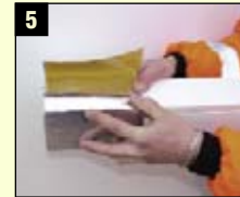
5 Check that the wrap fits comfortably around the trunking and introduce this combination into the opening
