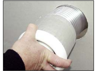
STEP 4: fit the Fireblok sleeve over the vent and fit to the ducting
