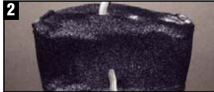
2 Insert cables through the cover. Hold onto the string to prevent the cover from falling into the cavity. Picture shows view from inside the cavity, where several cables have been inserted into the cover.
