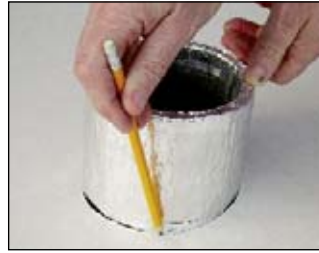
STEP 1: mark the outline for the Fireblok sleeve on the substrate
