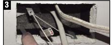
3 Continue to hold onto the string and cover, then push the fixing pins through the metal brackets and into the plasterboard.
