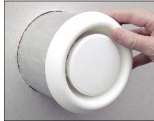
STEP 5: push the assembly back into the substrate until flush
