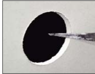
STEP 3: neatly cut out the hole with a padsaw and clean edges
