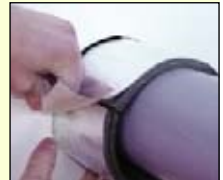
6 Whilst holding the wrap in place, remove the backing from the self-adhesive strip
