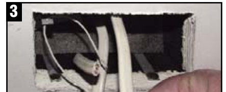
3 Continue to hold onto the string and cover, then push the fixing pins through the metal brackets and into the plasterboard. Afterwards, cut and remove the string.
