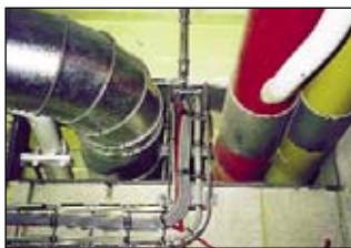
Pillows fitted into floor and ceiling service penetration areas. 38mm diameter wire mesh A is used to support pillows fixed with Envirograf® FB/C metal straps B
