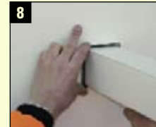
8 Finally, push the wrap into the opening until it is level with the surface
