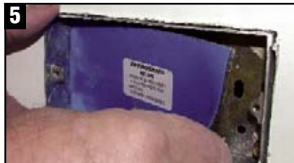
5 Insert the gasket into the metal box housing.
