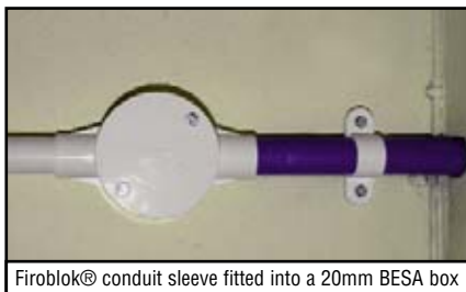
Fireblok® conduit sleeve fitted into a 20mm BESA box
