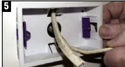
5 Insert cables into the socket housing.
