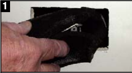
1 Compress the cover ready to insert into the aperture.
