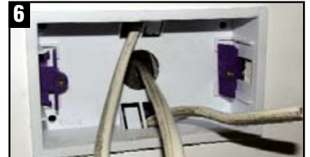
6 Connect cables to the socket front plate.
