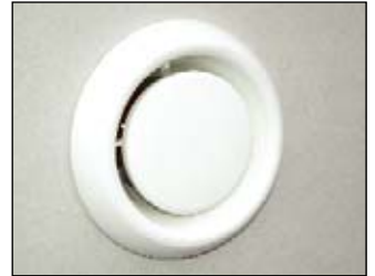
STEP 6: the finished vent with fire protection – a neatly finished job!
