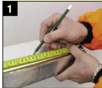
1 Measure the depth of the opening and mark this on the wrap. You cut off just what you need with no waste.
