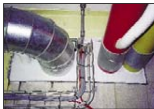
Pillows fitted into floor and ceiling service penetration areas. 38mm diameter wire mesh A is used to support pillows fixed with Envirograf® FB/C metal straps B
