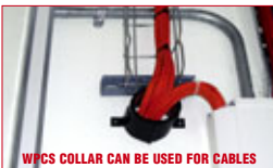
WPCS COLLAR CAN BE USED FOR CABLES
