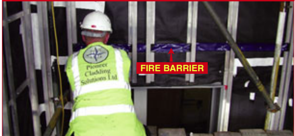
EXTERNAL FIRE BARRIER FITTED TO ESCAPE ROUTES
