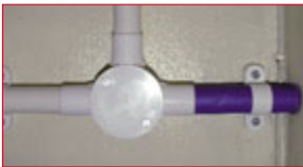
Fireblok® conduit sleeve fitted into a 25mm BESA box
