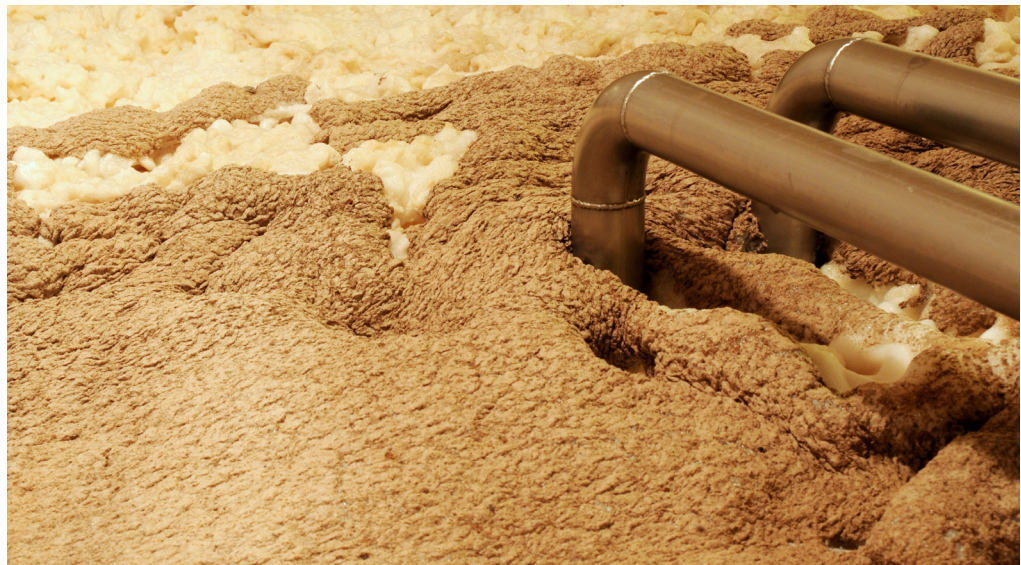
A fermenting cellar at a brewery demanding a pump to handle thick solid-laden slurry
