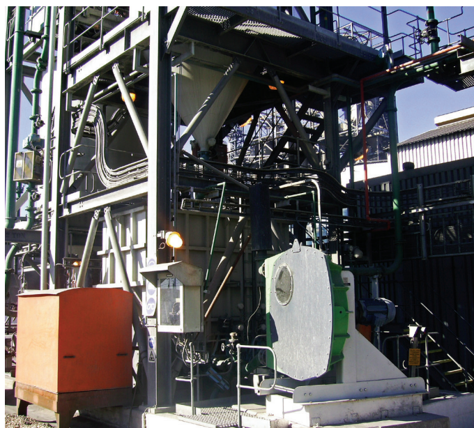
Left: A Verderflex pump circulating abrasive and corrosive lime slurry at Barston STW
