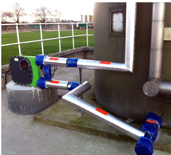
Left: A Verderflex pump circulating abrasive and corrosive lime slurry at Barston STW
