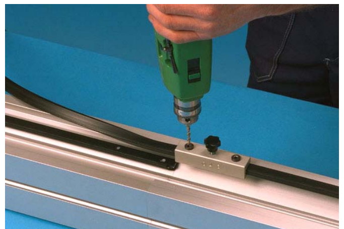
5 On the upper flange of the slide rail, use the drill fixture to drill two holes in the slide rail before it enters the XKCB N beam.
