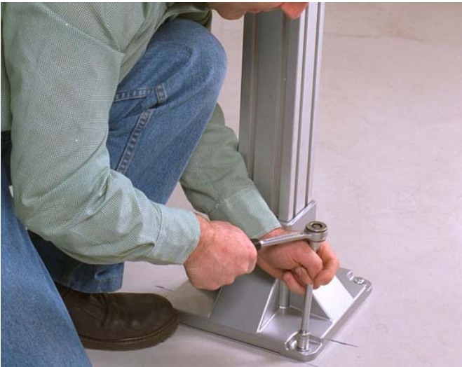
5 Fasten the foot to the floor.
