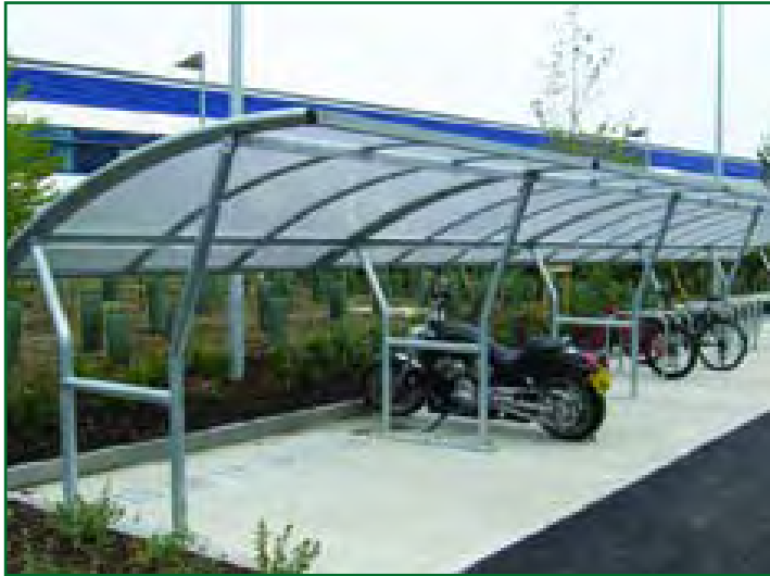
Galvanised frame, polycarbonate roof + extn bays
