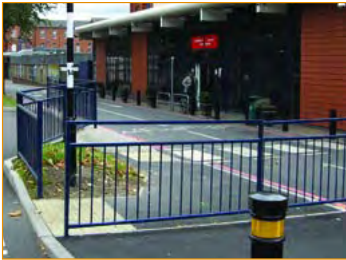
Pedestrian Guardrail with see through top
