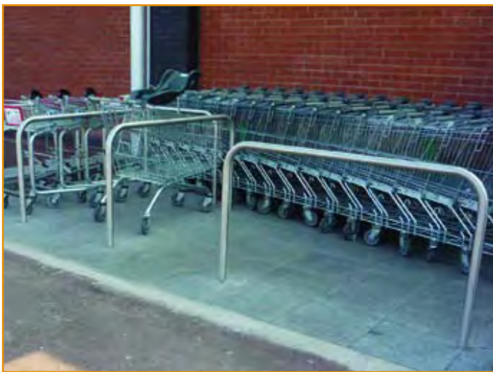
Special trolley bay, stainless steel finish
