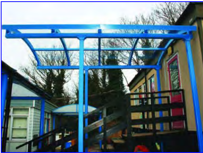
Bespoke walkway with adjusted and lengthened legs
