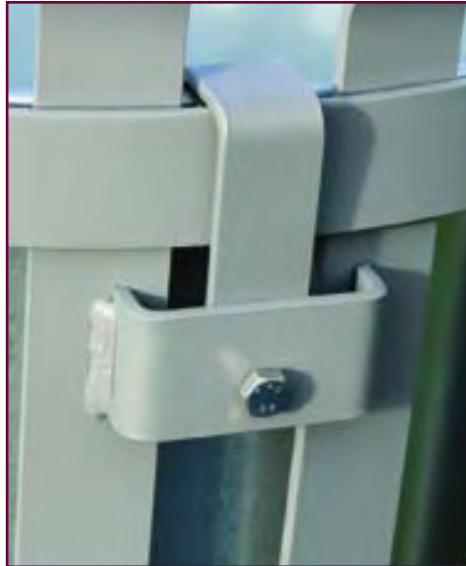
Locking latch to secure liner
