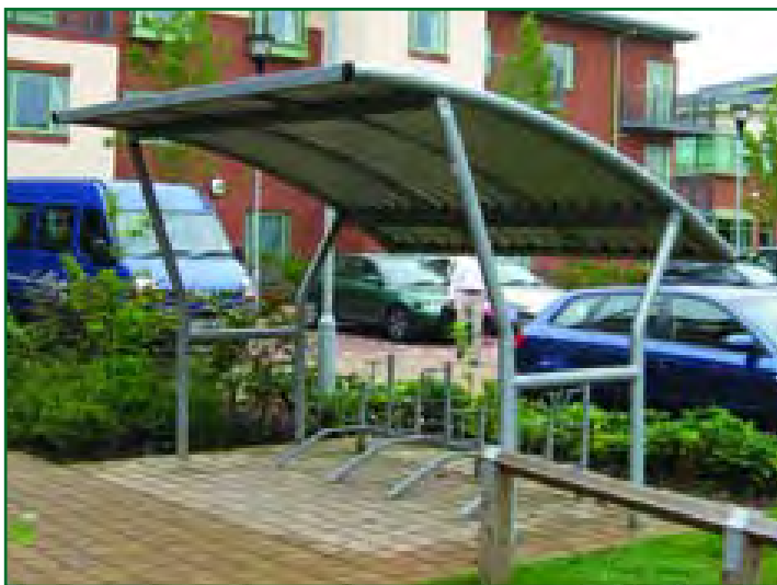
Galvanised frame and roof
