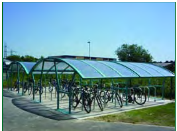
Galvanised & painted frame, polycarbonate roof + extn bays
