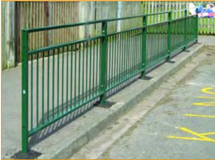
Pedestrian Guardrail with see through top
