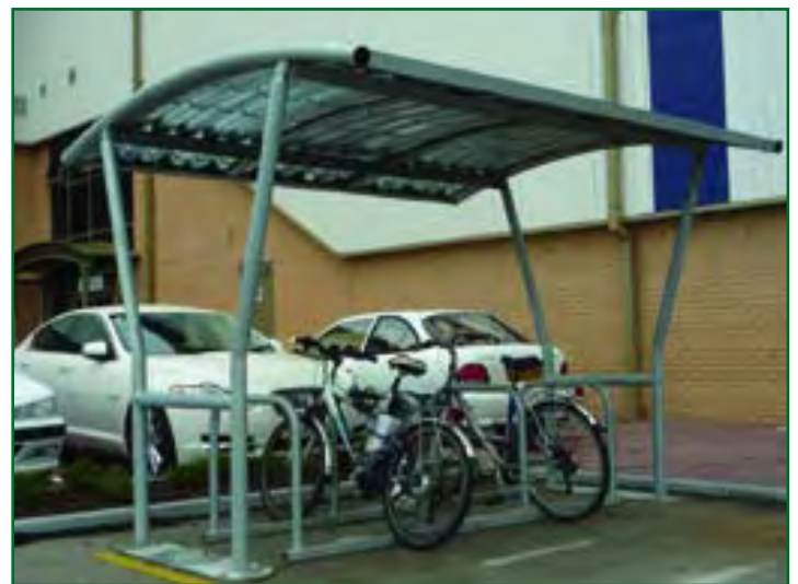
Galvanised frame & roof
