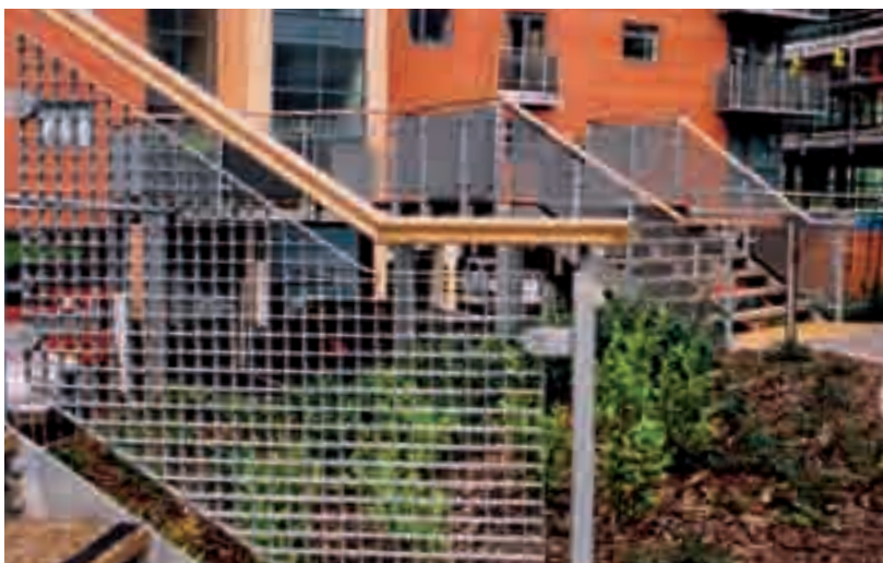
Staircase infill panels, Leeds
