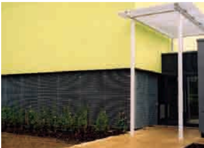
Cladding panels, Essex
