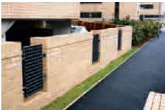
Architectural car park infills in Leeds
