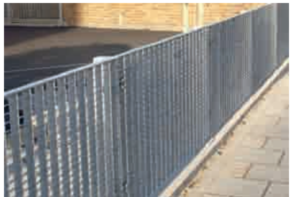
Perimeter fencing, London
