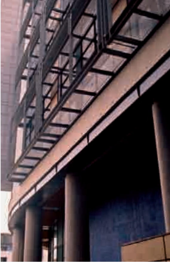
Brise soleil walkway panels, Edinburgh
