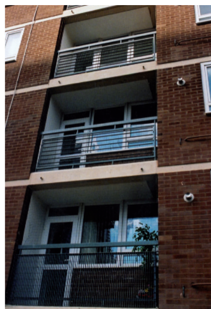
Balcony infills in Liverpool
