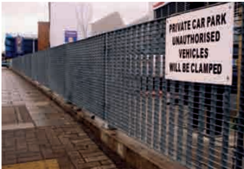
Fencing, Ilford in London
