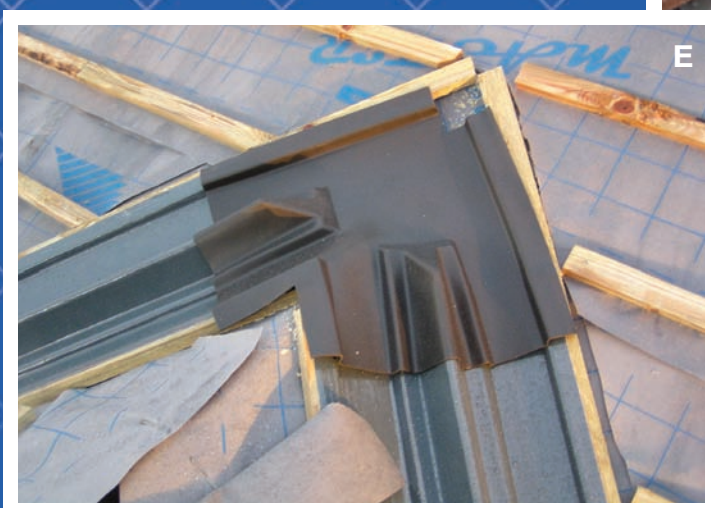
E. The top closure 90 or 75 should be fixed in position over the two joining FILON V-Flow DF valley troughs.
