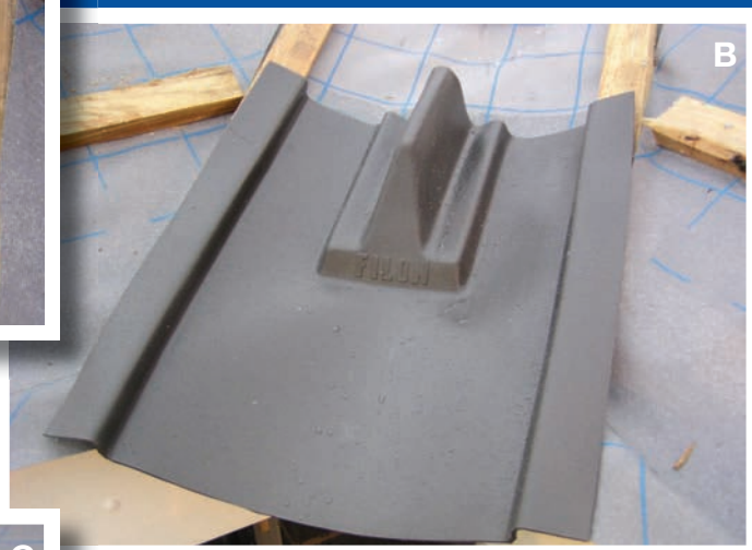
B. The eaves closure piece is placed over the support – a flexible packing piece is used to support the sides of the closure if the battens do not extend to the fascia.
