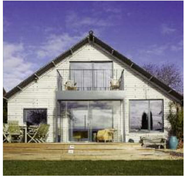
Profile 3, Ensworth Coastal House, Hampshire
