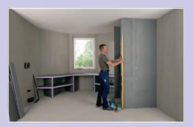
The shower partition wall is finished. Prior to laying the tiles, all of the board joints outside the shower must be filled with JACKOBOARD glass fibre tape.
