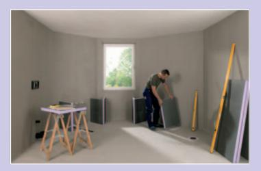
The construction board elements are glued to the wall and floor to provide the substructure for the washstand.
