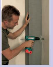
The angle element JACKOBOARD Canto is ideal for quickly cladding pipes; it can be installed both vertically and horizontally. JACKOBOARD anchors spaced 80 cm apart at the most are plugged onto the angle element and bolted to fasten it.
