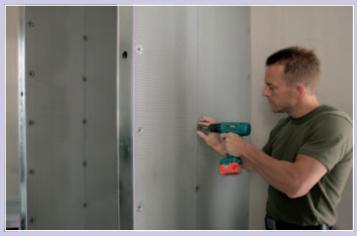
JACKOBOARD Plano is fixed using suitable metal screws (5 per m<sup>2</sup>) and JACKOBOARD insulation board discs.
