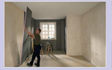
JACKOBOARD Plano is aligned to the floor at an angle, pressed onto the substrate and straightened with the help of a spirit level.
