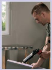
JACKOBOARD Plano is measured and cut to size. Assembly adhesive is applied to the top edges.
