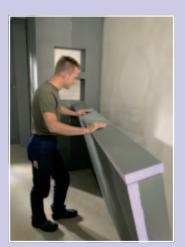
Once they have been measured and cut to size, the individual construction boards are fixed with assembly adhesive. Individual construction board ribs can be integrated for additional stability. The built niche with shelves and the tray design can be glued to the wall and floor using assembly adhesive.
