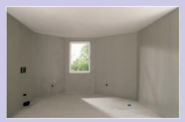
The bare shell of the bathroom. The walls have been plastered, the screed laid. The bathroom can now be individually designed with the help of JACKOBOARD construction boards.
