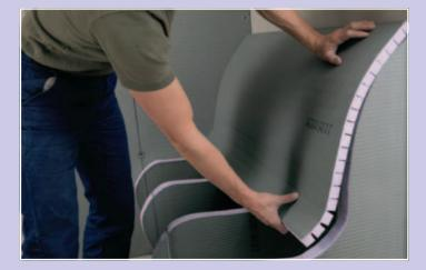
The slotted surface of JACKOBOARD Flexo makes it easy to adjust it to exactly the shape of the substructure. The creative construction board is positioned with the slotted side facing down and fixed with assembly adhesive. For easier installation, the creative construction board can also be fixed with a few wooden screws. All joints and visible top edges then need to be covered with JACKOBOARD glass fibre tape or sealing tape.
