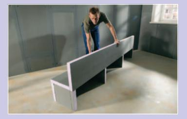
To create the bath panelling, a supporting structure is built using 50 mm JACKOBOARD Plano construction boards and glued with assembly adhesive.
