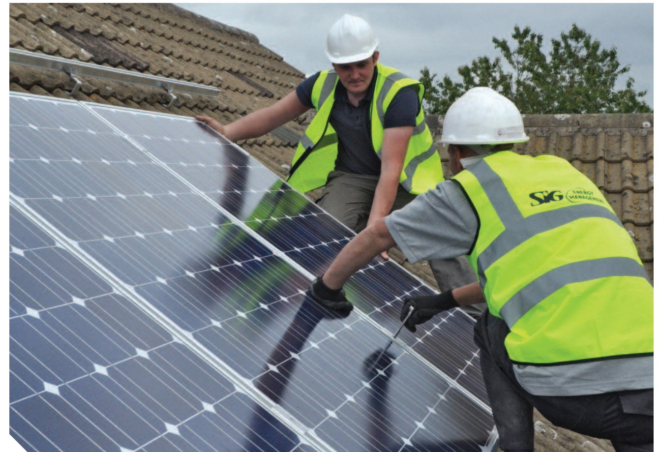
Solar Panel Installation
