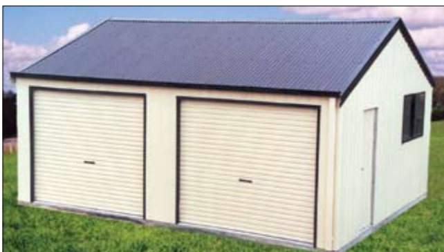
Double Garage with roller doors on gutter side
