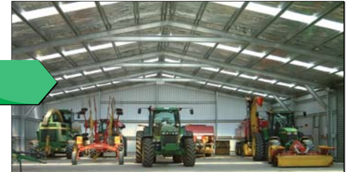
Internal view of Industrial building
