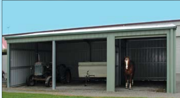
3 bay Farm Shed with roller door in one bay
