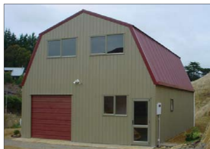
Quaker Barn with 1 roller door 22
