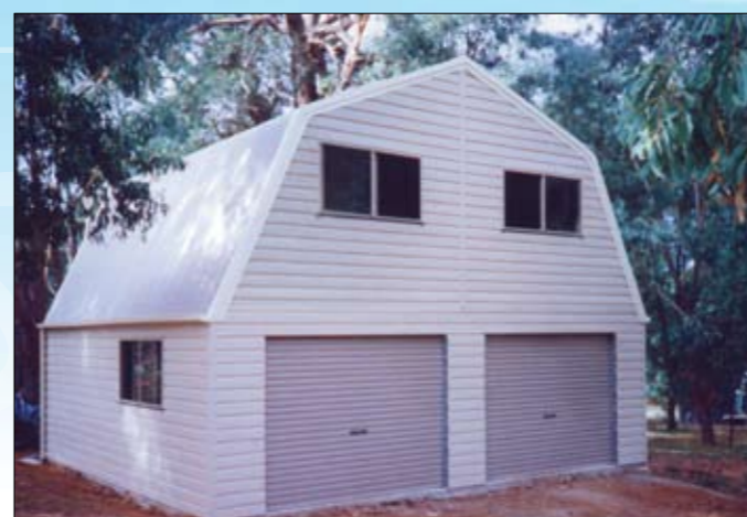
Quaker Barn with 2 roller doors 20
