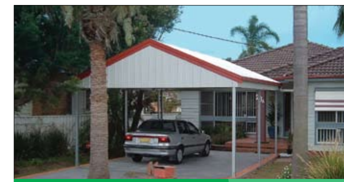
Pitched roof Carport
