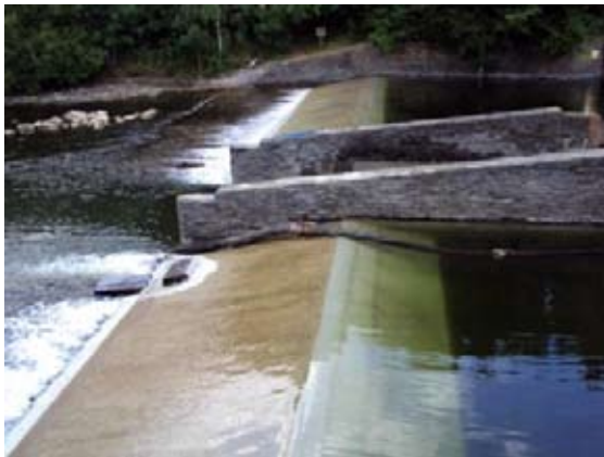
Rockbond Underwater Mortar used to repair the bridge and weir at Newby, Ulverston
