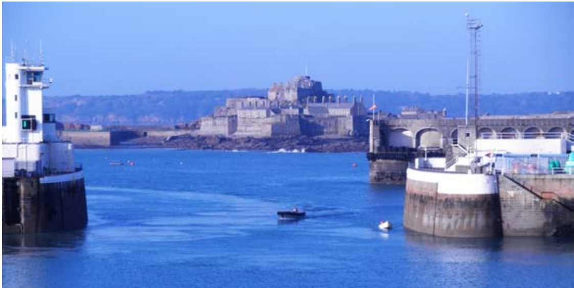
Rockbond Underwater Mortar use to protect concrete piers against scour attack at the Queen Elizabeth Ferry at Jersey Port, Channel Islands.
