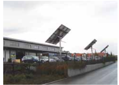
These solar panels that are mounted on poles can be scanned from the back to minimize reflection.
