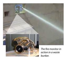
"The fire monitor can also be handed manually with a joystick. This is necessary so that the system can be overruled by firemen. In case a fire should break out firemen can not only use the fire monitor to help them extinguish the fire. Thermal imaging cameras like the FLIR A615 can also see through smoke. This means that the PYROsmart system will help firemen to see where the fire is and where they are spraying the water, through the smoke."
