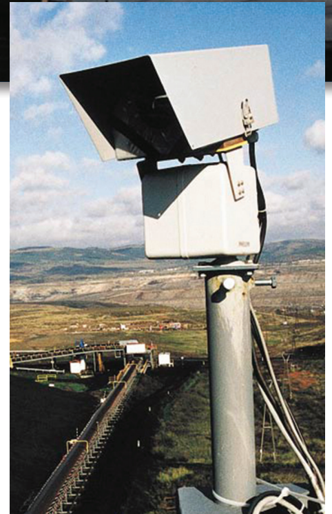
The FLIR Systems thermal imaging camera mounted on a mast over the coal piles of the Nástup Mines Cooperation in the Czech Republic.
