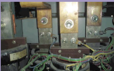
BURNT WIRE FOR POWER METER AND VOLTAGE & AMP METER
