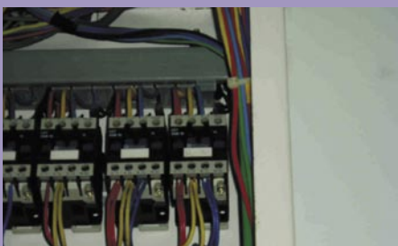
LOOSE CONNECTION CAUSED HEAT BUILD UP IN LIGHTING CONTACTOR
