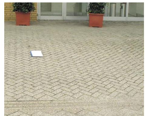
severe district heating pipe leak spotted by FLIR Systems ThermoCAM™ S65
