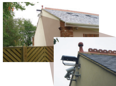
These two FLIR SR-313 thermal imaging cameras have adjacent fields of view, together they cover a large part of the surrounding fields.
