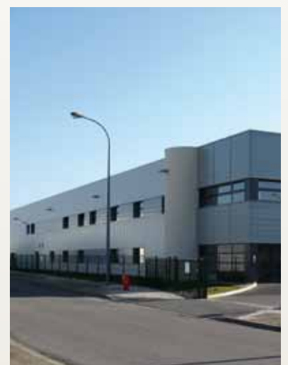
CEAT Electronique's main factory and repair center in Longvic, France
