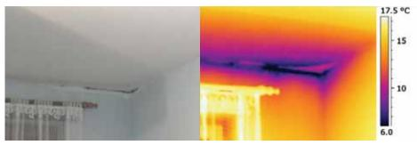
This corner of the room has been damaged due to water leakage. If nothing is done the water damage might threaten the structural integrity of the building.
