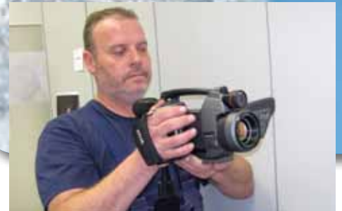
Maintenance engineer Thorsten Krämer uses the FLIR P620 to inspect a fuse cabinet.
