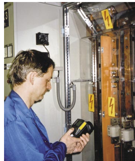
Jan Heyselbergs uses the ThermaCAM™ E2 for electrical inspections
