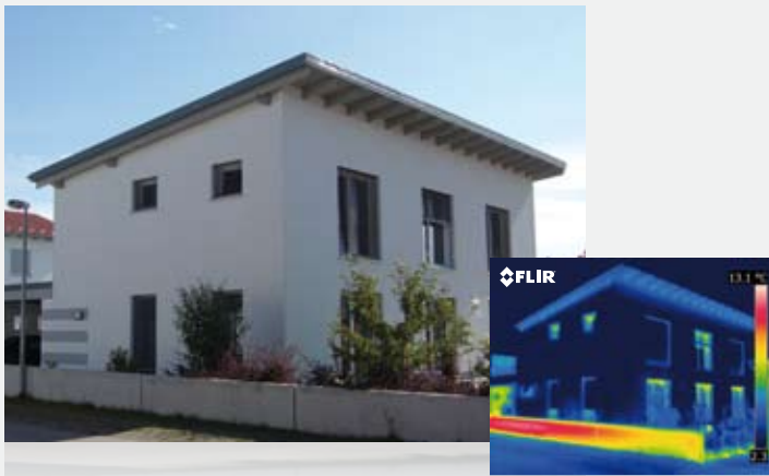
Infrared image shows insulation quality of a low energy house
