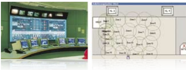
Figure 7. Control room for waste pile processing, and screen capture of the zone monitoring layout, which uses a FLIR IR camera on a pan-tilt mount for fire hazard warning.
