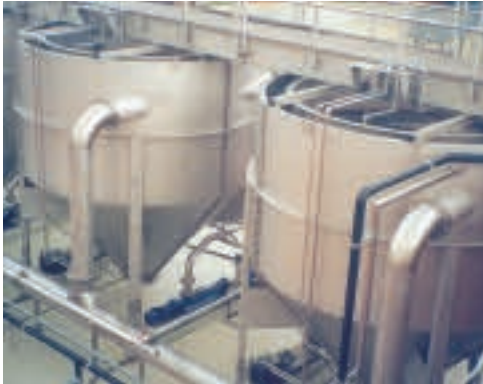
A pair of ROTAMAT® Circular Grit Traps HRSF
