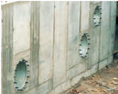
Flush with the wall
