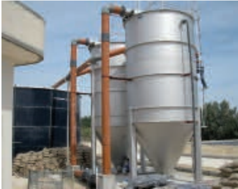
CONTIFLOW® Sandfilter CFSF, stainless steel tank design
