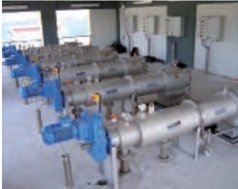
STRAINPRESS® – continuous pressurised coarse material separation
