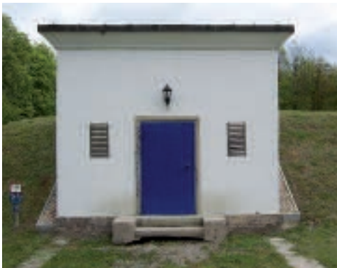
Drinking water reservoir with HUBER equipment
