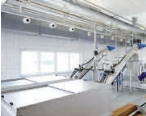
ROTAMAT® Rotary Drum Fine Screen Ro 2 with up to 3 m screen basket diameter
