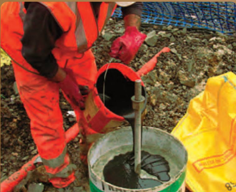
Applying bearing material to pile caps for precast concrete units
