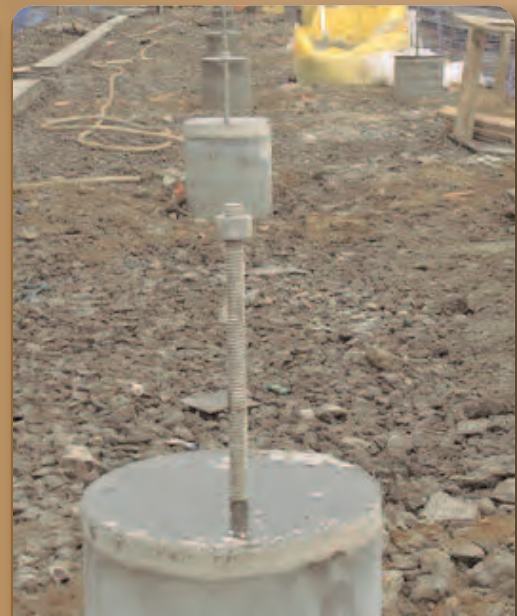
Finished pile caps for precast concrete units
