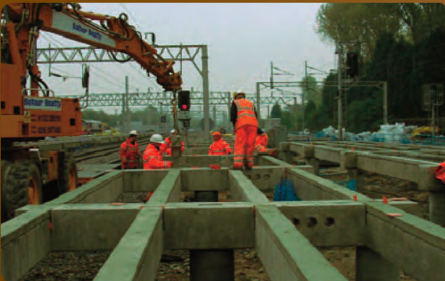
Installing longitudinal beams into the crosshead pockets
