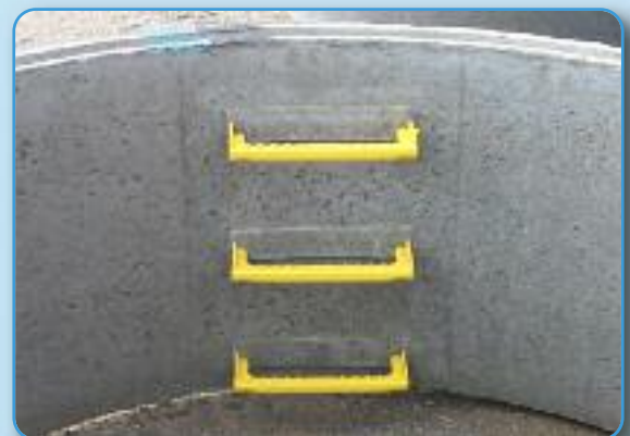
Double steps in chamber section
